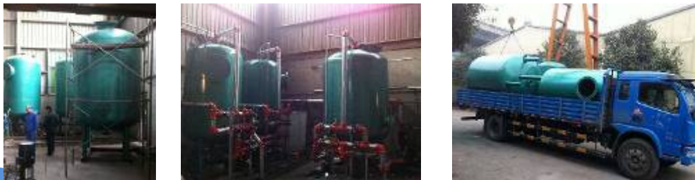
40m³/h Water Softener + Multi-media filter system
