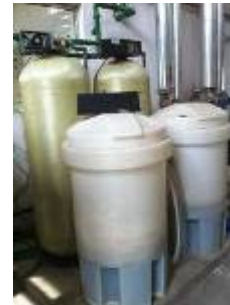
40m³/h Water Softener + Multi-media filter system
