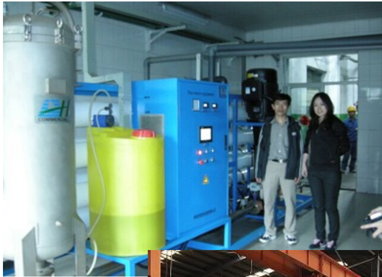
Vietnam client visiting our pure water treatment plant
