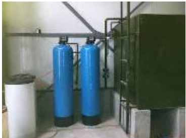
40m³/h Water Softener + Multi-media filter system
