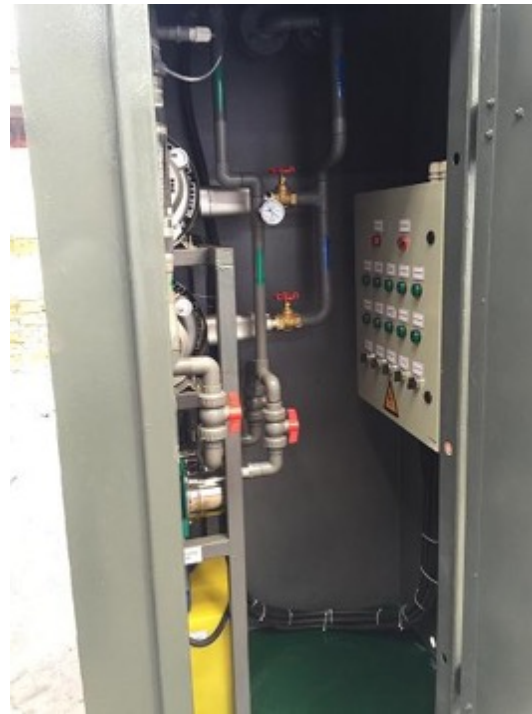
Compact control cabinet inside with pump sets & blower sets
