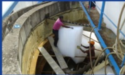
INSTALLATION IN SIDE THE CLARIFIERS
