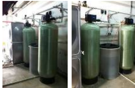
40m³/h Water Softener + Multi-media filter system
