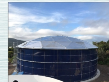
Landfill leachate treatment
