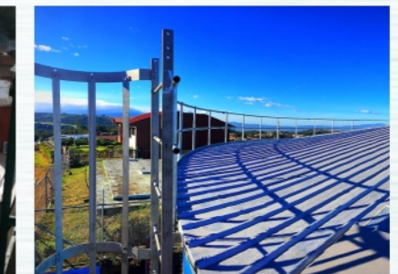
Aluminum Trough Deck Roof
