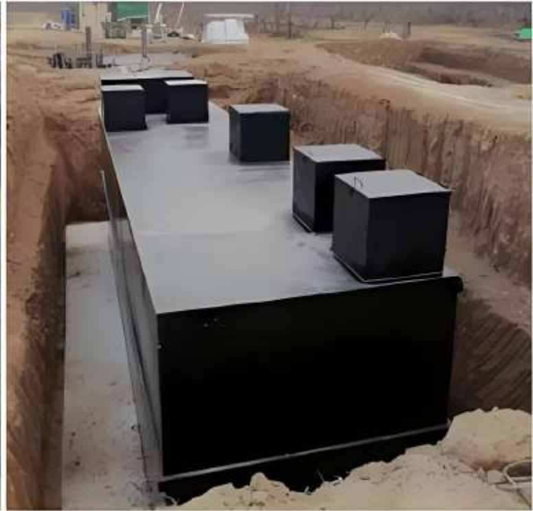
APS 20 tons/day Sewage treatment plant On ground Installation
