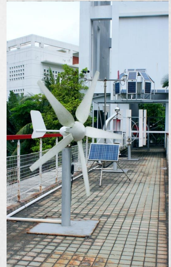
Solar & Wind Hybrid Pumping System Operational Testing & Data Collection
