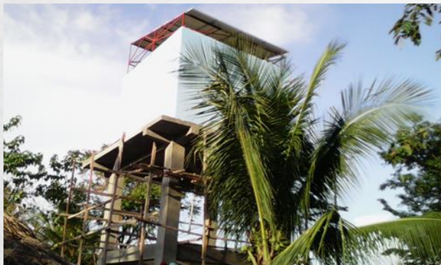
Solar array installed above the water tower
