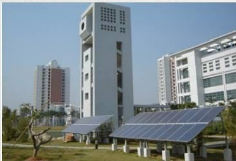
Solar Pump Operational Testing & Data Collection
