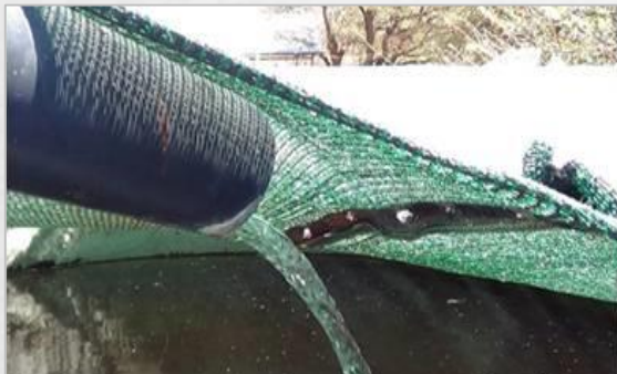
Water pipe installed
