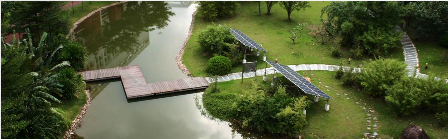
Solar Pumping System Operational Testing & Data Collection
