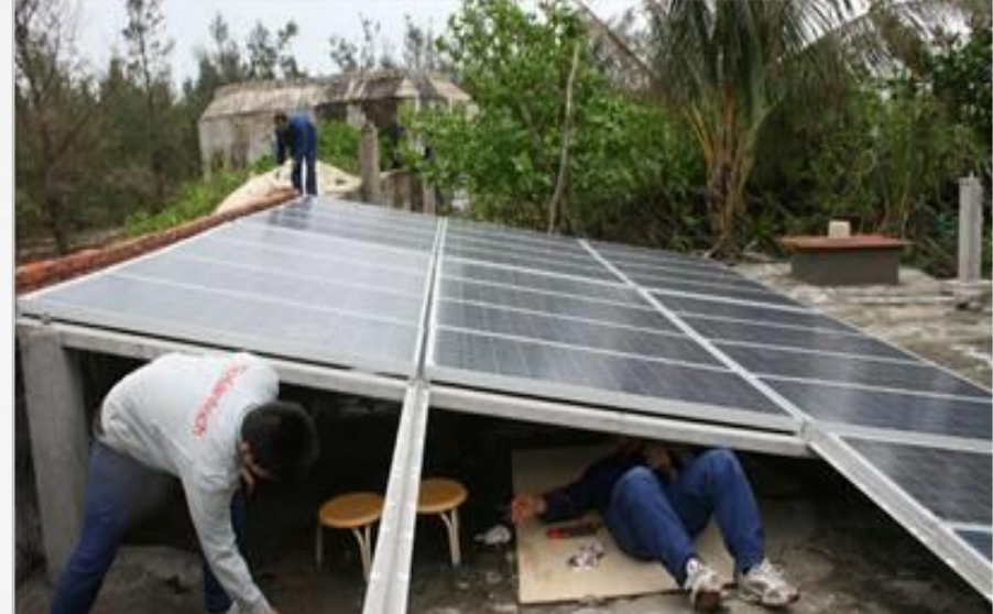
Install solar array
