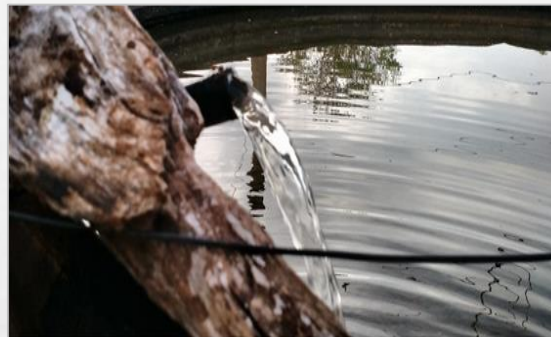
Water flow injecting into reservoir
