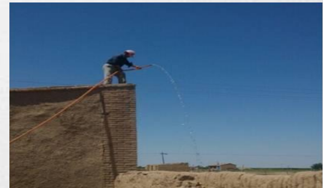
Water pipe installed
