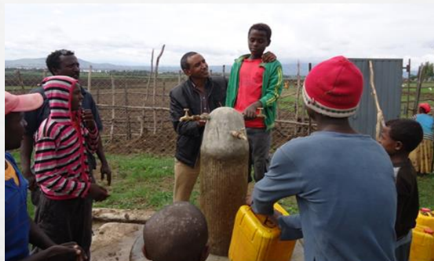
Water faucet installed
