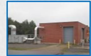
Clean Water Treatment
